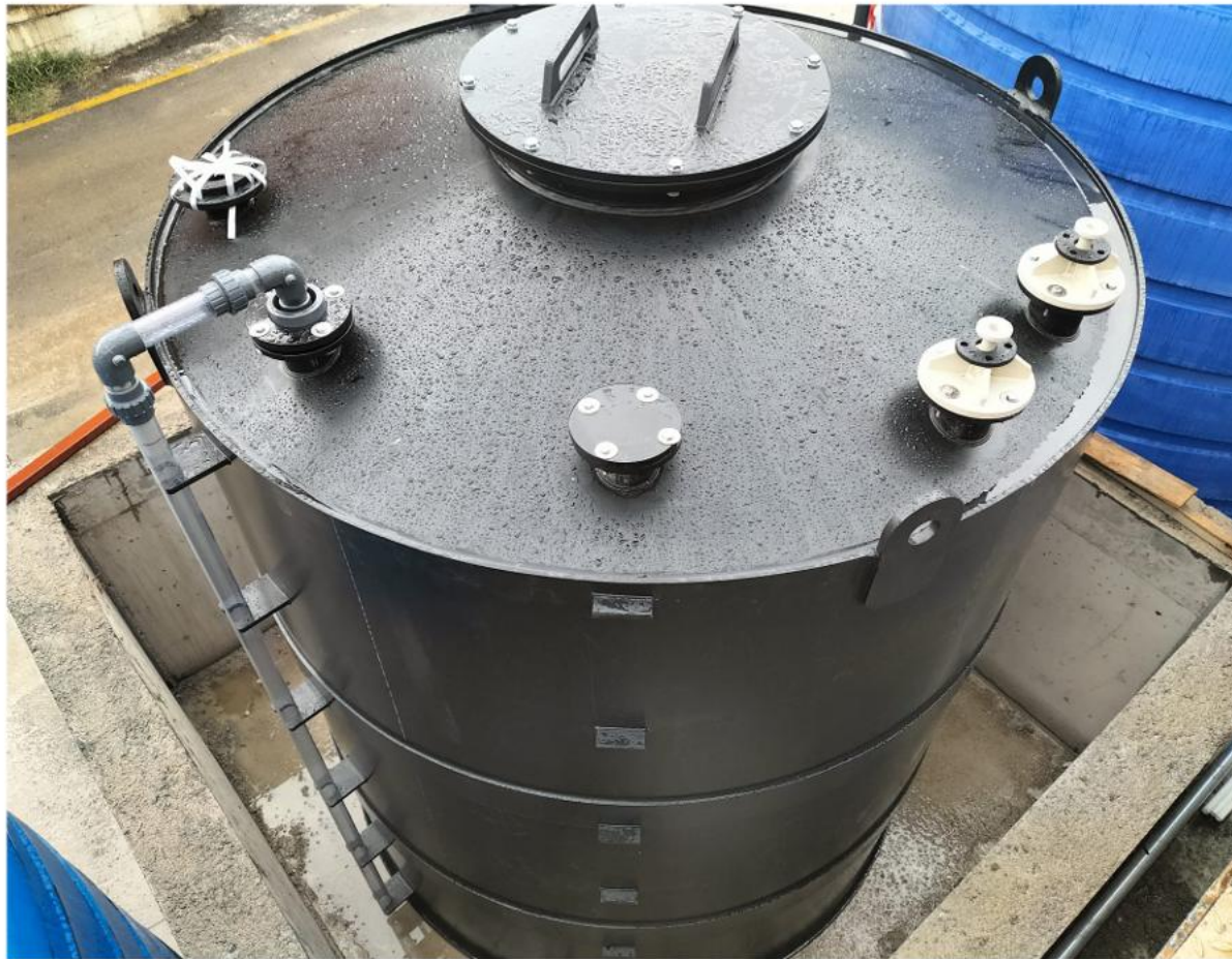
HDPE Chemical Treatment Transfer Tank, Egypt
